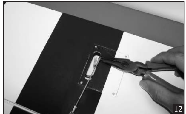
Insert the nylon clasp to the metal rod.
